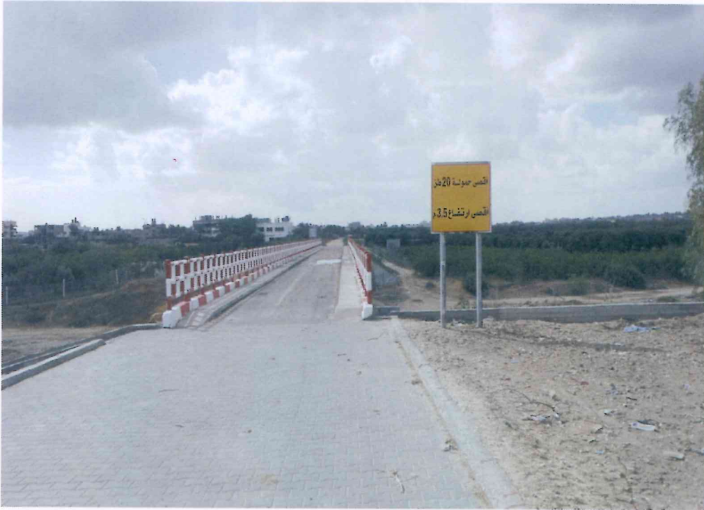
AL Sikka Bridge (Before Damaged)
